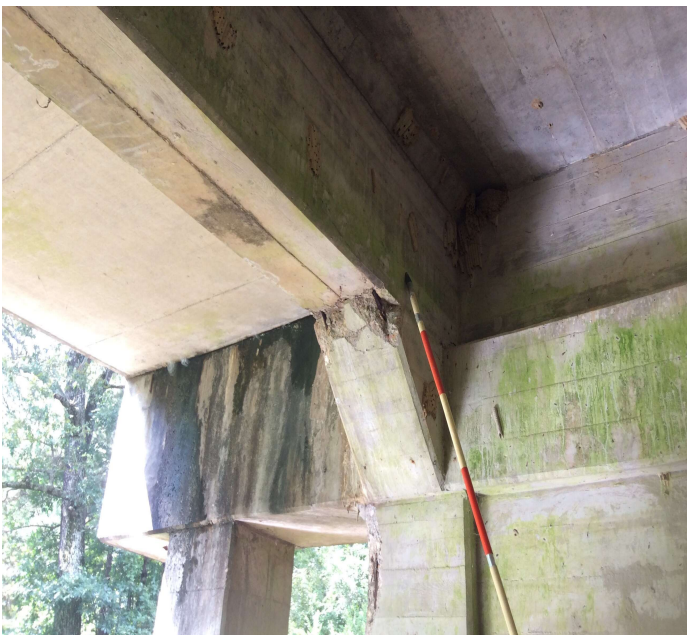
PHOTO 1 Description Span 2, girder 3, Bt. 2, exposed rebar at haunch of the girder.
