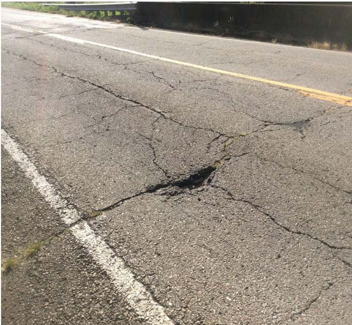
PHOTO 1 Description Potholes
