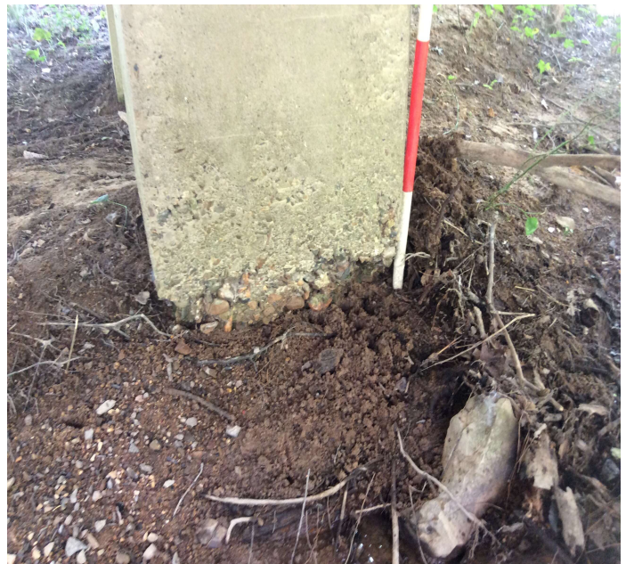
PHOTO 2 Description Bt. 2, column 2, severe abrasion.
