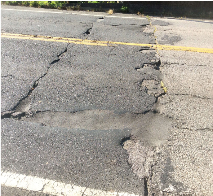
PHOTO 1 Description Approach roadway settlement
