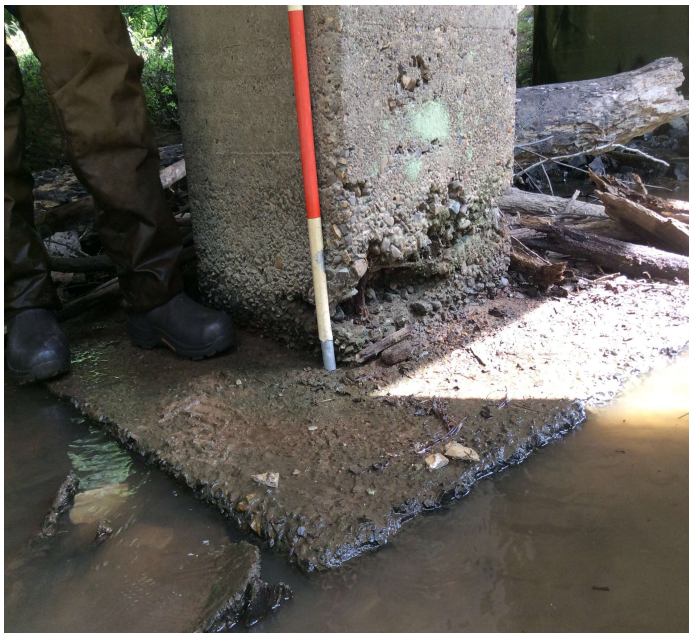
PHOTO 1 Description Bt. 2, column 3, severe abrasion exposing the rebar.
